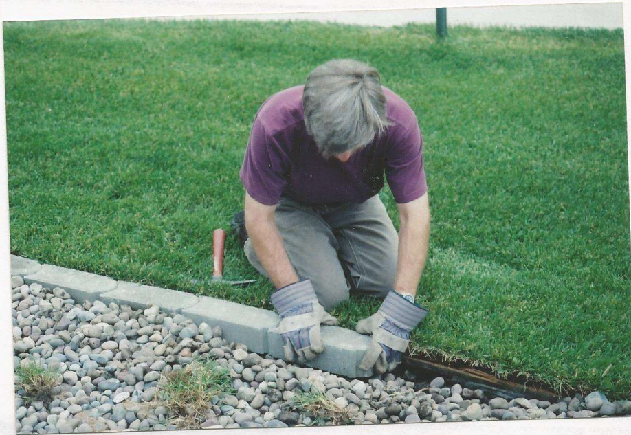
Steve DeLay setting concrete edging
