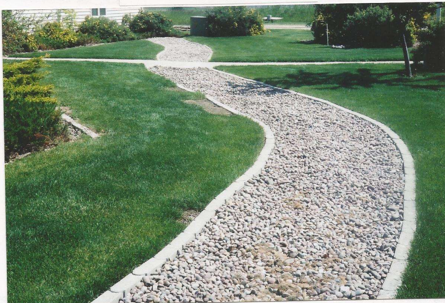
Replacing cedar edging w/concrete June 2004
