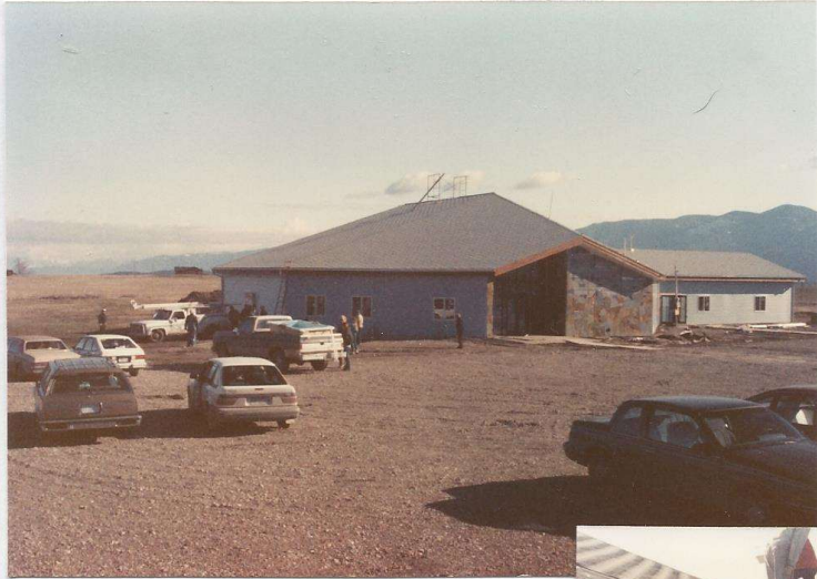
Putting up the Steeple 1989
