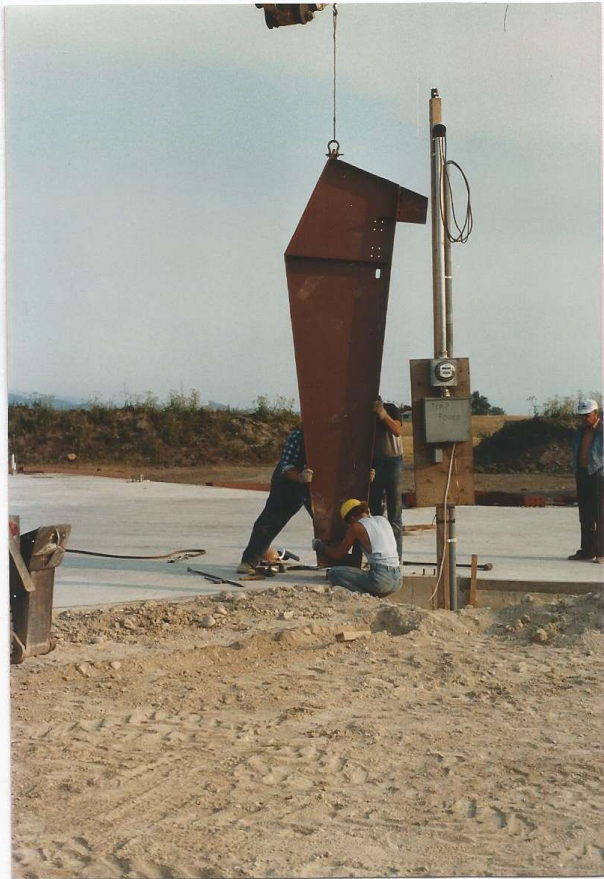
MORE STEEL WORK September 2, 1988
