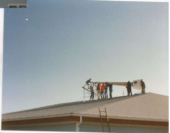
April 8, 1989 Hoisting the steeple in place.
