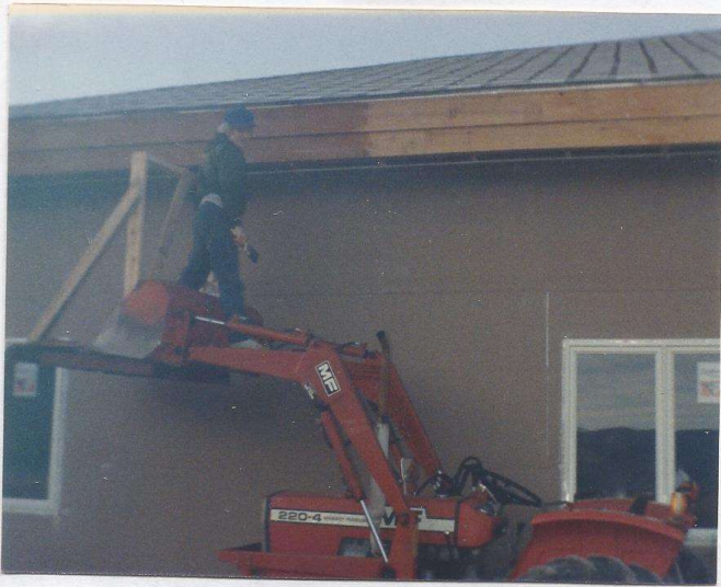
October, 1988 Alice DeLay staining fascia board.
